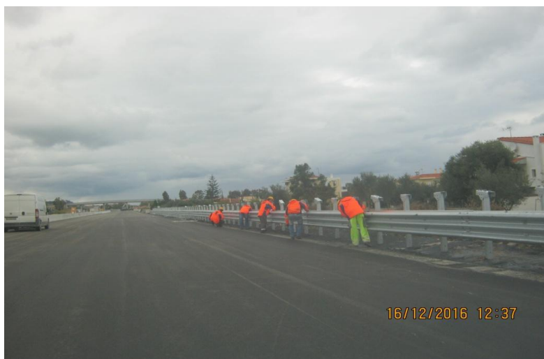
Steel safety barrier installation at k.p. 22+000 to k.p. 29+500
