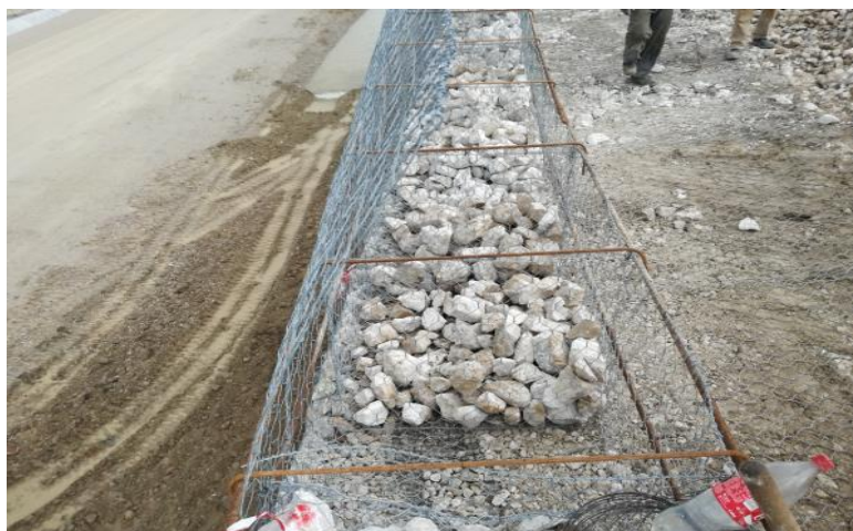
R289 – Construction of the reinforced soil wall
