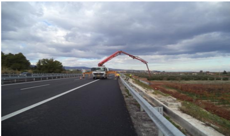
Concreting of drainage ditches at k.p. 10+000 to k.p. 14+000
