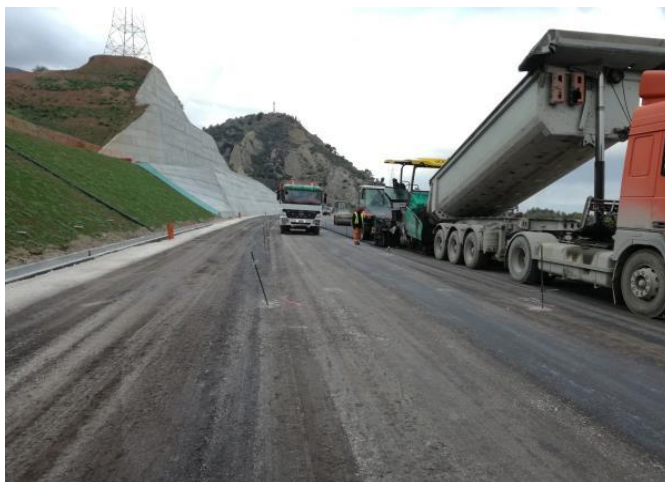
Asphalt works at k.p. 47+350 to k.p. 47+500
