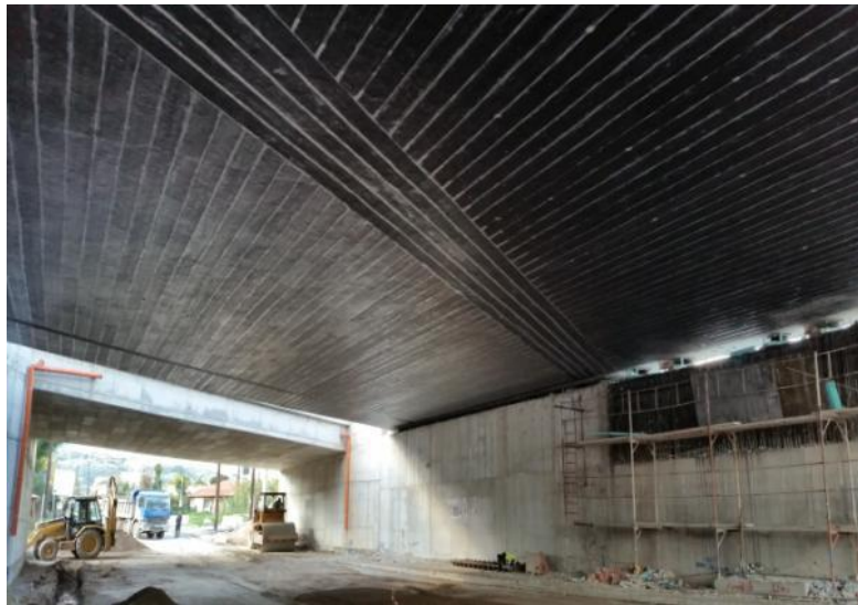
Completion of FRP strips installation at K305
