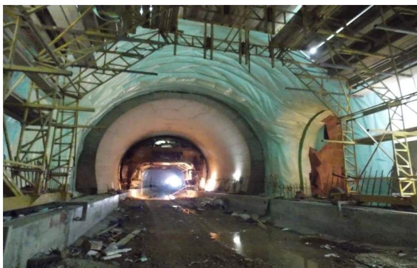
Waterproofing & reinforcement placement at Platanos tunnel- West portal/South bore
