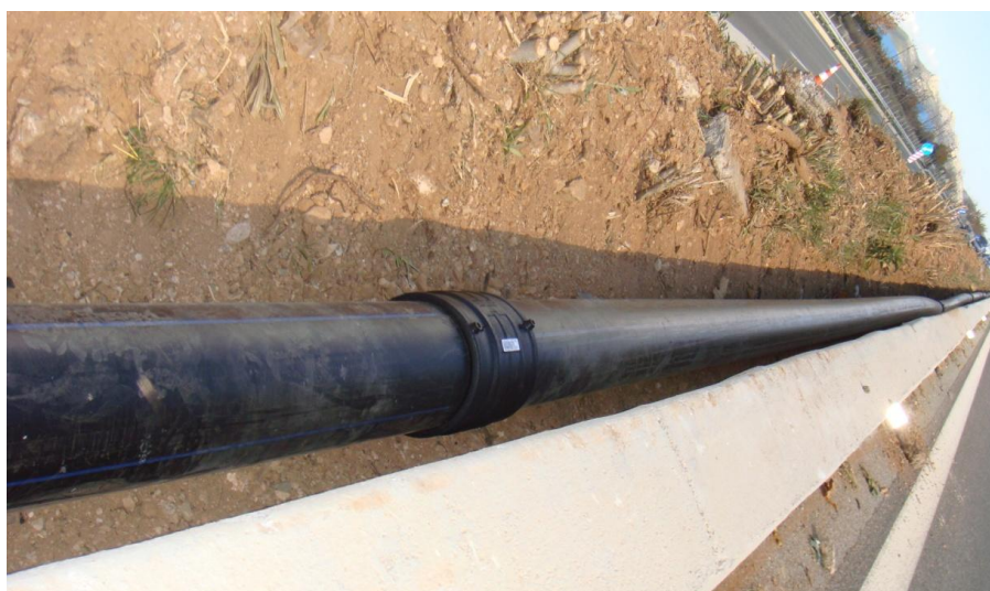
Installation of irrigation pipes
