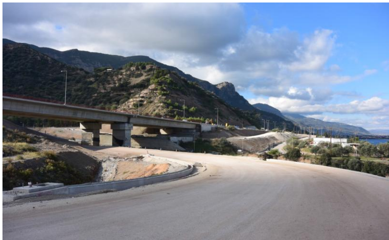
Construction of CDF platform towards Kalavryta
