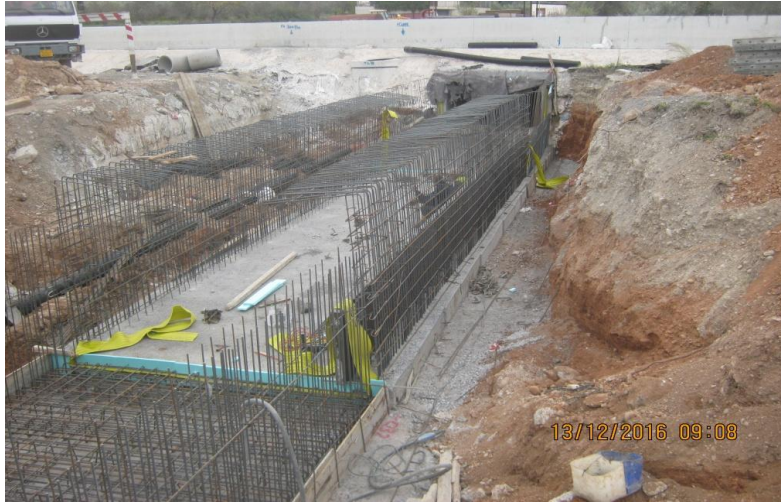
L218 – Construction of box culvert
