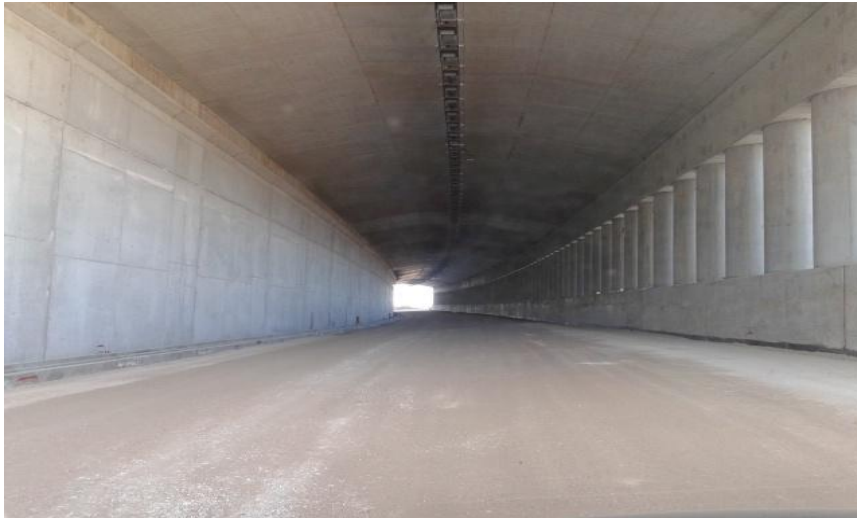
C004 – Construction of CDF layer
